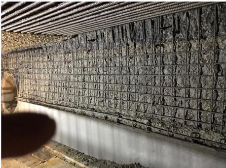
As part of a major £16 million upgrade of Eastbourne Wastewater Treatment Works, Intercrete concrete repair materials were chosen to refurbish an underground inlet chamber at the plant. Almost 140 tonnes of Intercrete 4801 was applied over a six month period by specialist asset maintenance contractor, Concrete Repairs Limited.
